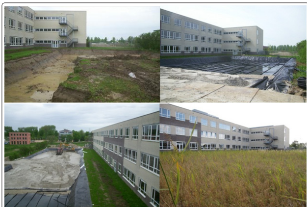
Figure 1: Construction of a Constructed Wetland
