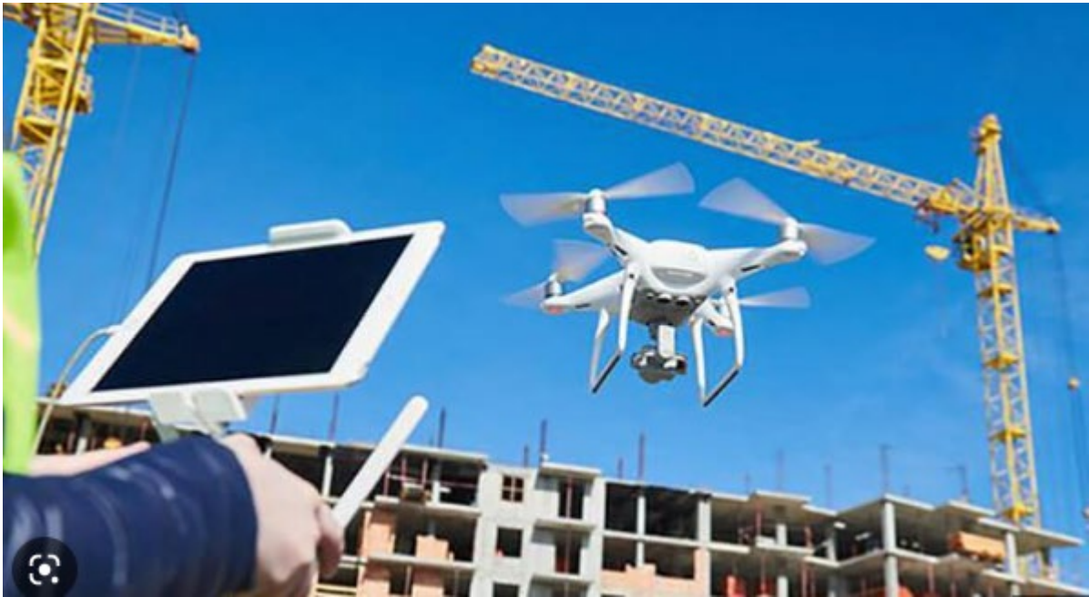
Figure 4: Building construction monitoring by a drone
