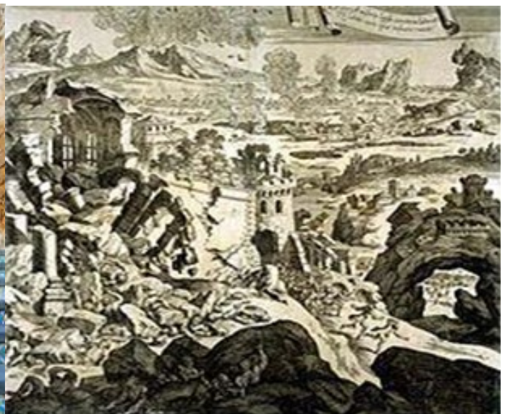
Figure 5: The Lisbon earthquake
