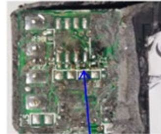
Replacing with a new capacitor
