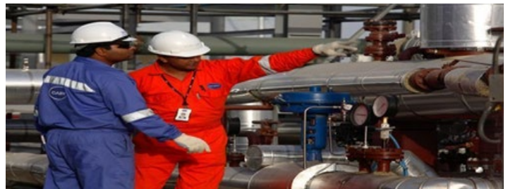
Figure 6: Workers at gas distribution station [36].
