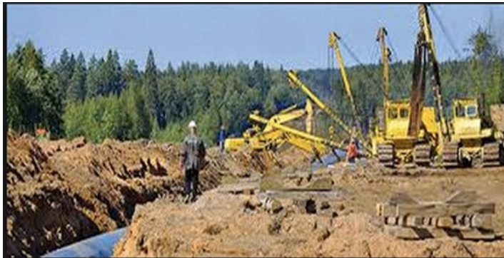
Figure 4: Pipeline installation project activity (FEMA 2013)
