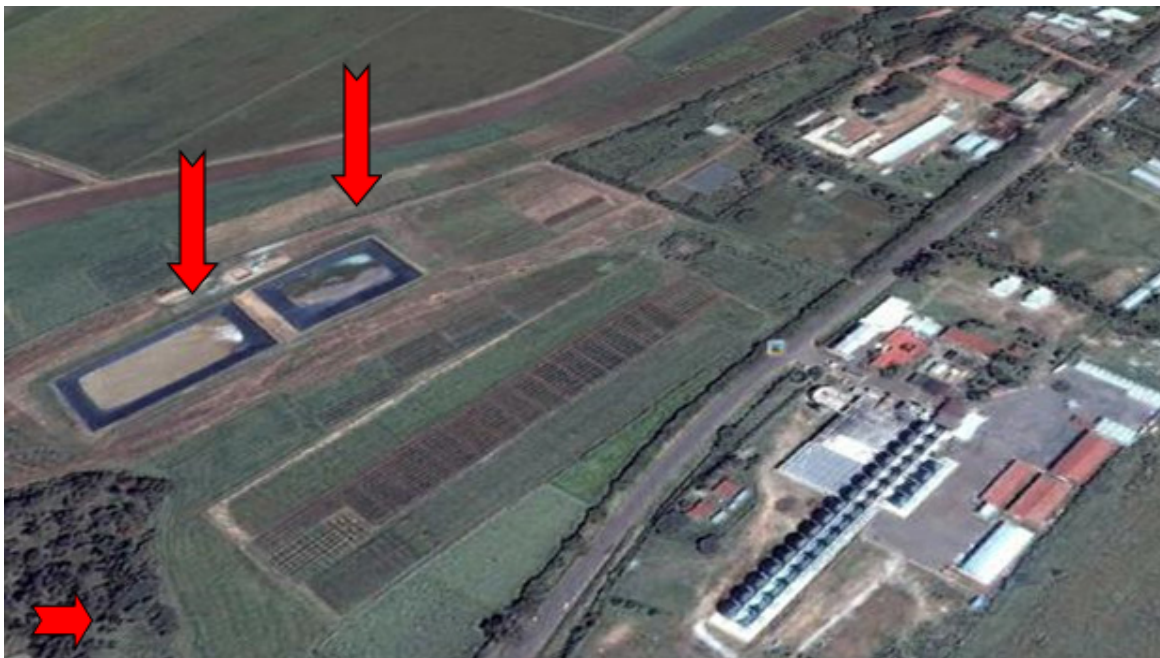
Figure 2: The KARC's previous structure of irrigation water reservoir ponds.
