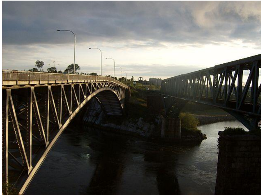
Figure 2: Reversing Falls Bridge (Left)
