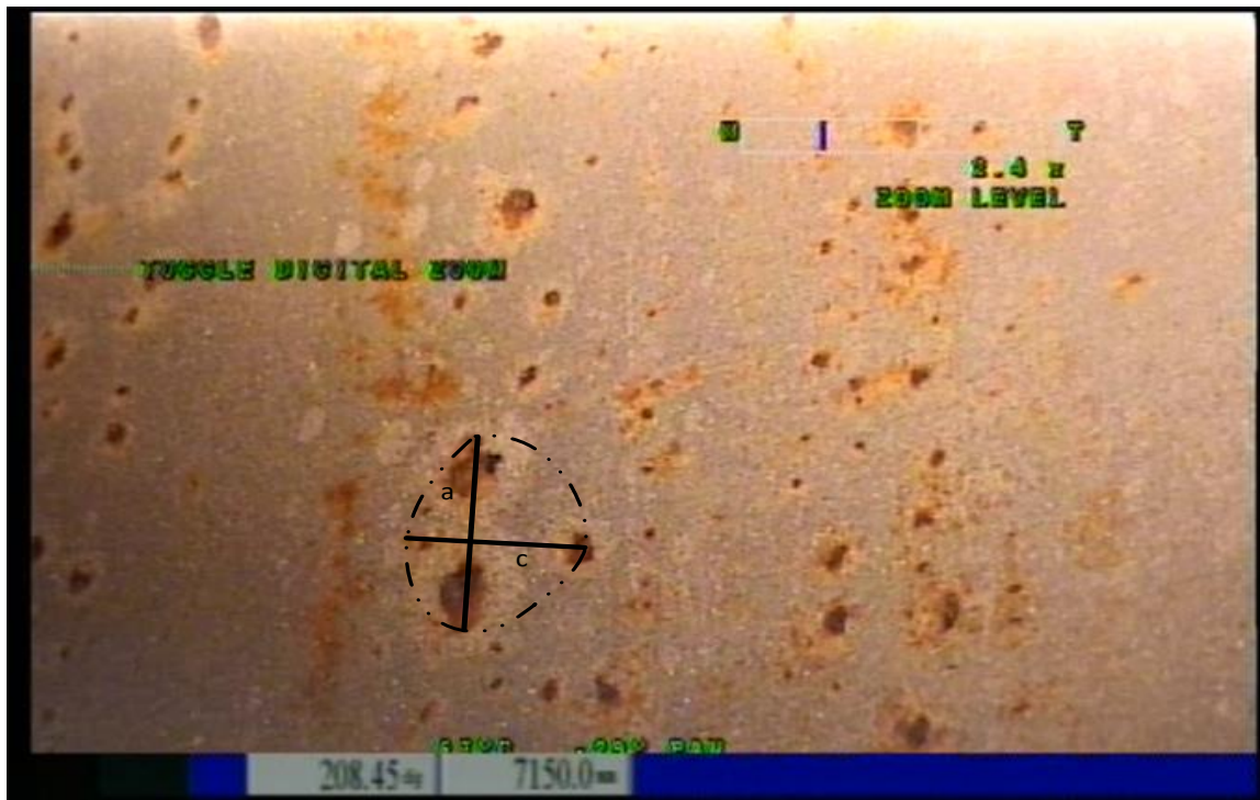
Figure 7: Cluster of Defects on the Inner Surface of the Reactor Vessel
