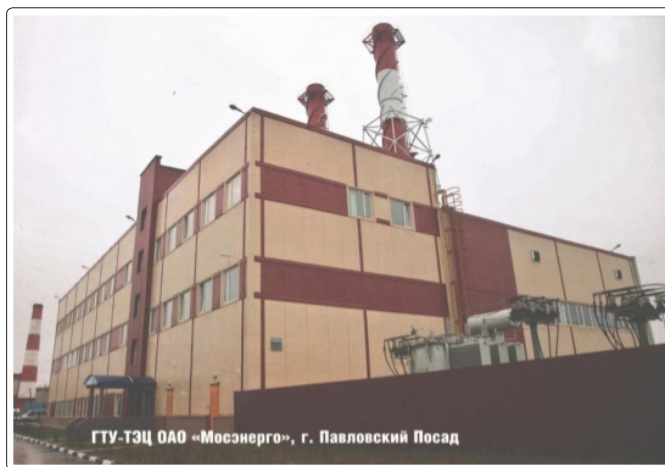
Figure 1: Gas turbine power station
