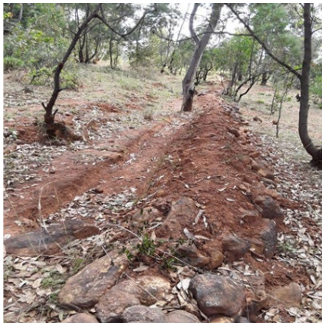
Figure 9: Stone-faced soil bund, Hadiya (Source; field survey)
