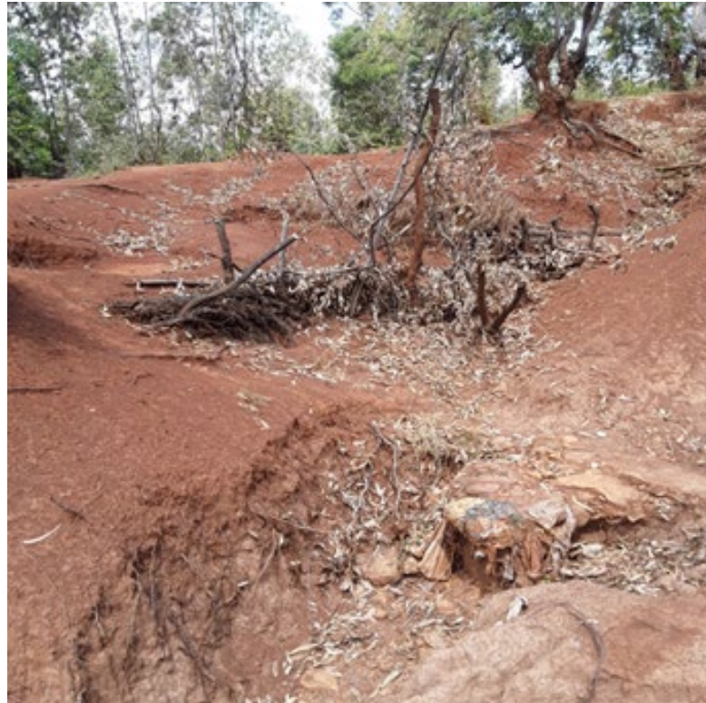
Figure 10: Brushwood check dam, Hadiya (Source; field survey)
