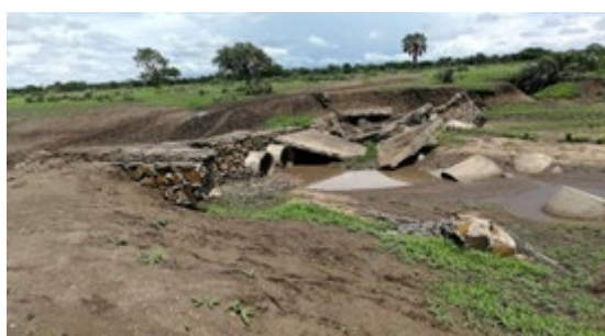
Plate 1: A Bridge Damaged by Floods at Chindoko Villagw, T/A Ngabu
